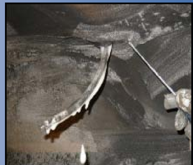
HYDROPHILLIC GROUT AT WORK
