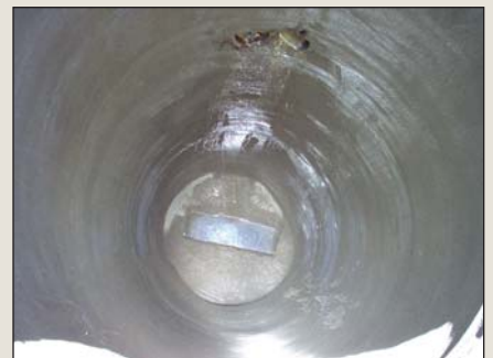
Above: Manhole before lining. Below: Manhole relined.
