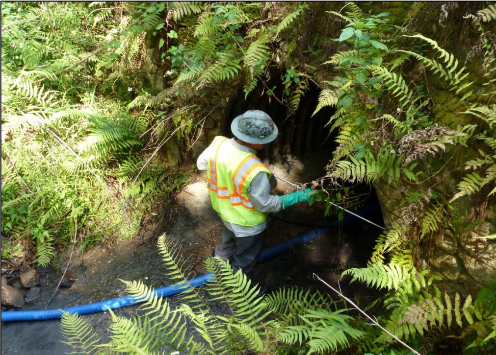
THE PIPE & CULVERT REPAIR CONNECTION
