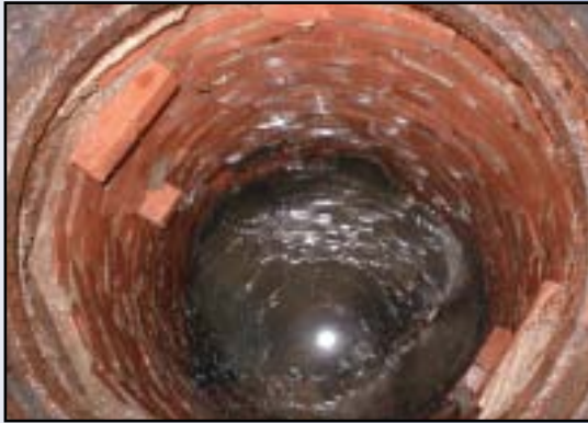
Brick manhole cleaned and ready for Cement Liner
