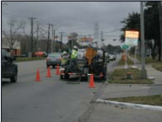
Manhole crew mixing material for application of Reliner MSP cement liner.
