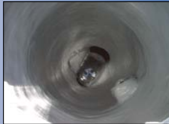
Manhole has been rehabilitated using RelinerMSP cement and StandardShield epoxy coating.
